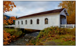
K305 Covered Bridge
